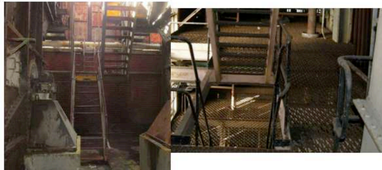
IMAGE OF SEVERELY CORRODED MEZZANINE STAIRCASE AND FLOORING TO BE ALL BE DEMOLISHED
