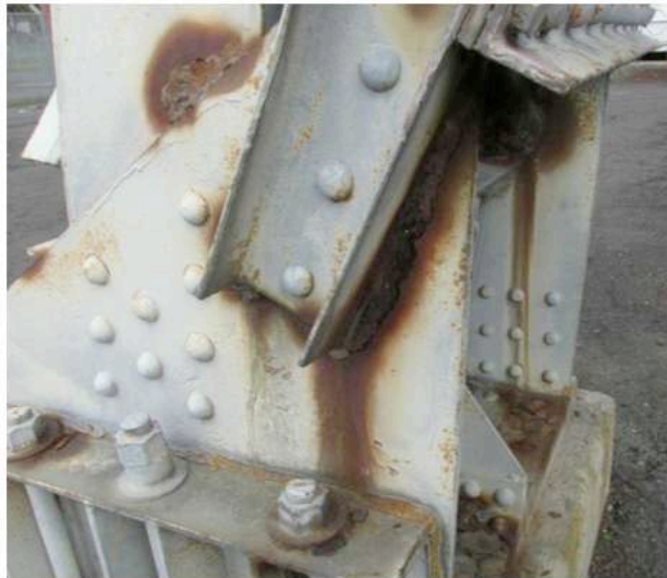
IMAGE OF STRUCTURAL STEEL SUPPORTS TO BE SAND-BLASTED AND REPAINTED
