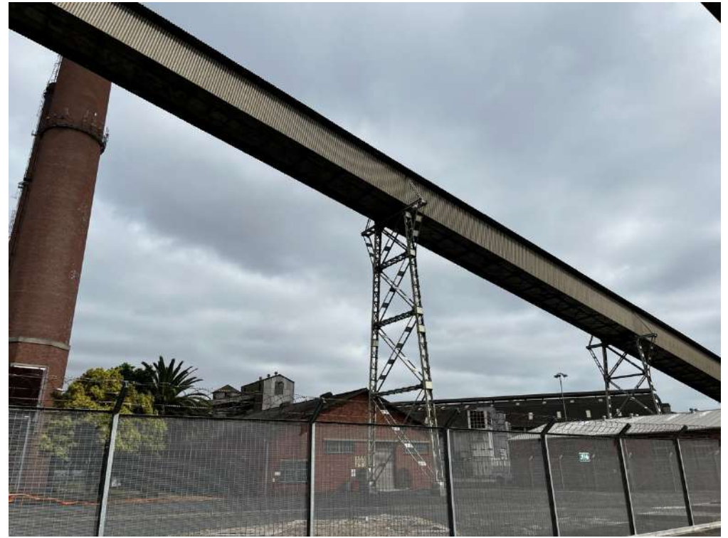
Figure 34: Coal Conveyor structure running between Boiler House and Junction Houses (Hearth, 2025)
