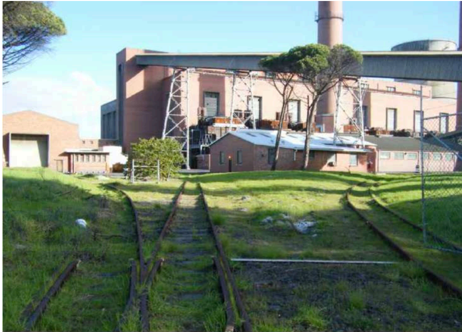
Figure 46: Photo of turbine hall, boiler house and coal conveyor and store showing railway tracks leading through the site (Sandra van der Merwe, 2008) – these railway tracks are no longer in situ as can be seen in Figure 28: Turbine Hall, Boiler House, chimney stacks, store 2 and coal conveyor with ash bunker to the right. (Hearth Heritage, 2025)
