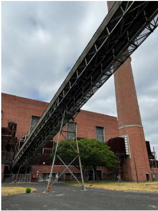
Figure 36: Ash Conveyor and Ash Plant (Hearth, 2025)
