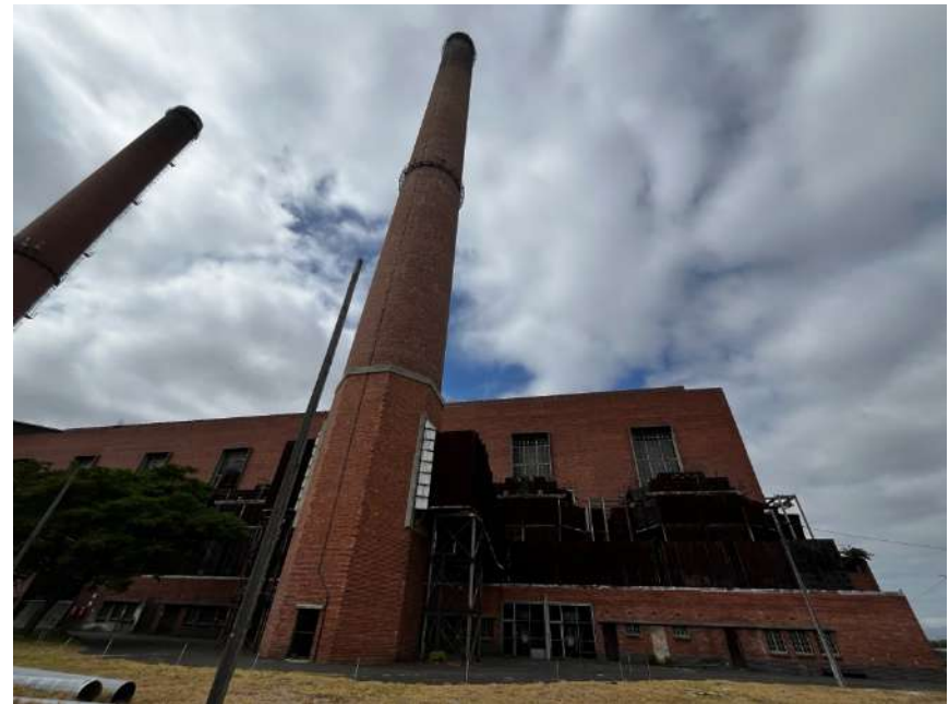
Figure 31: Boiler house with ash collectors on top and chimney stacks with turbine hall behind
