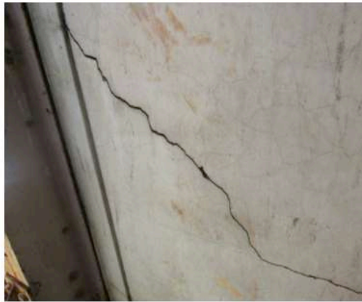
IMAGE OF MASONRY CRACKED WALL ON THE NORTH-WEST AND NORTH-EAST CORNER TO BE REPAIRED AND REPLASTERED
