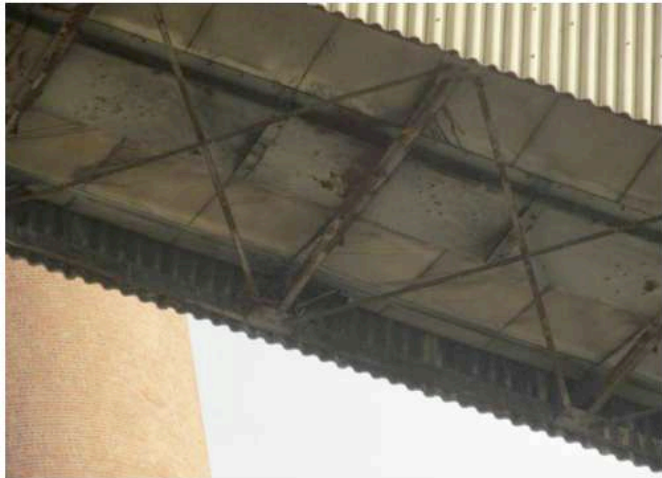
IMAGE OF SURFACE CORROSION OF STRUCTURAL STEEL MEMBERS UNDER COAL CONVEYOR TO BE SAND-BLASTED AND REPAINTED
