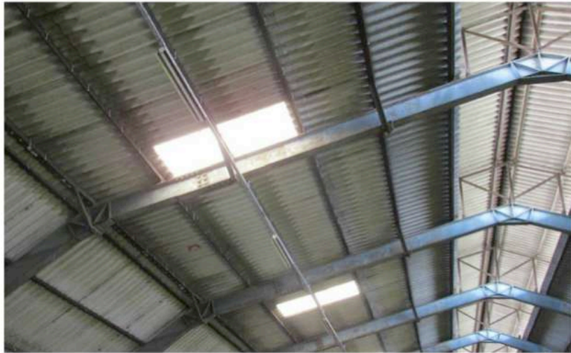
IMAGE OF ROOF STRUCTURAL STEEL MEMBERS TO BE SAND-BLASTED AND REPAINTED
