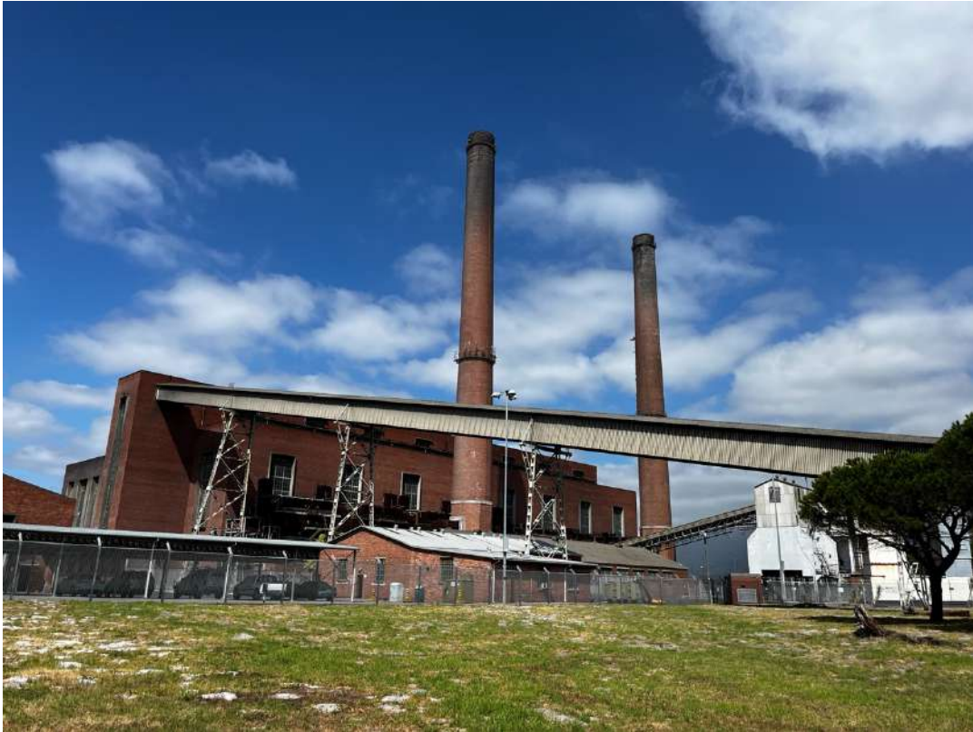
Figure 28: Turbine Hall, Boiler House, chimney stacks, store 2 and coal conveyor with ash bunker to the right.
